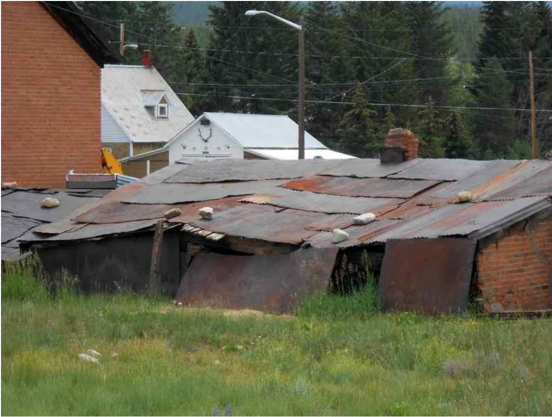
Picture 12: Various colors of weathered metal roofing.
