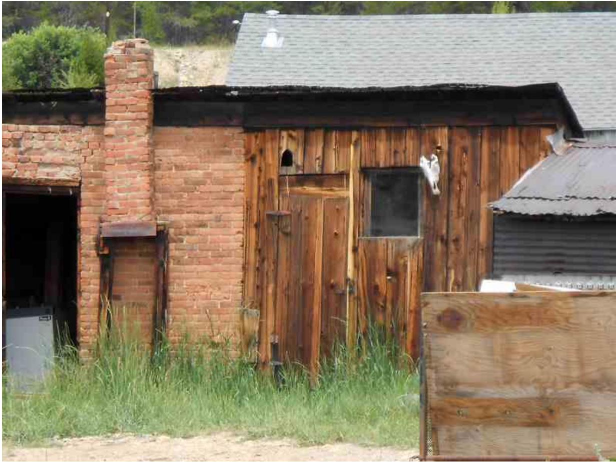
Picture 7: Orange siding along with brick. Note the chimney on a stand.
