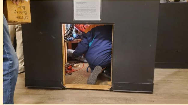
Photo 7: Working on wiring under the layout-2024
