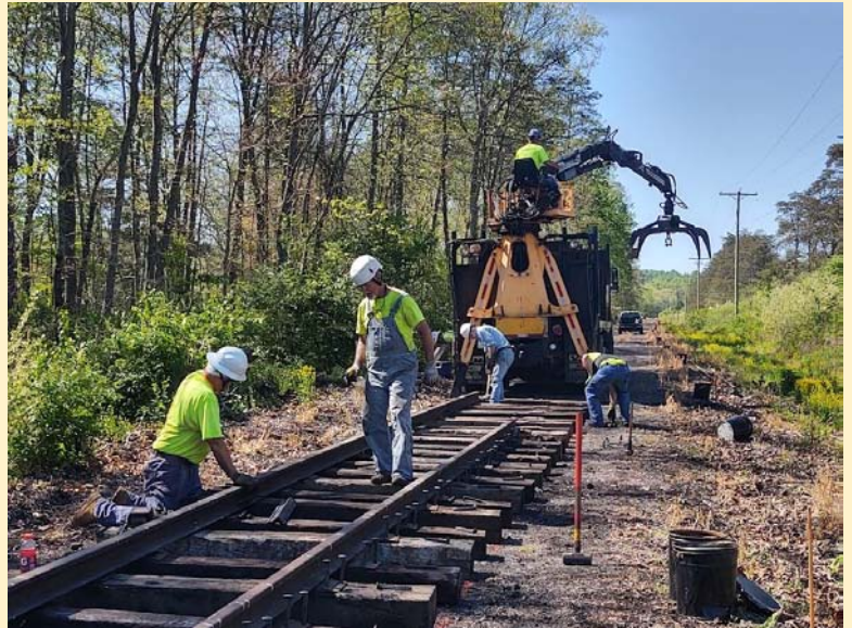
Making up joints south of 475 - May 2nd (Dave Johnson photo)
