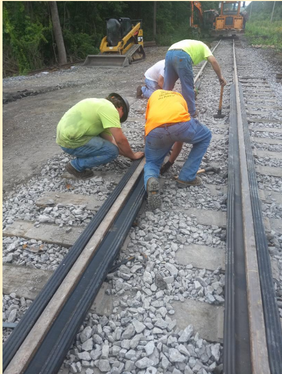
Installing rubber strips - Aug 6 th (G. Tucker photo)
