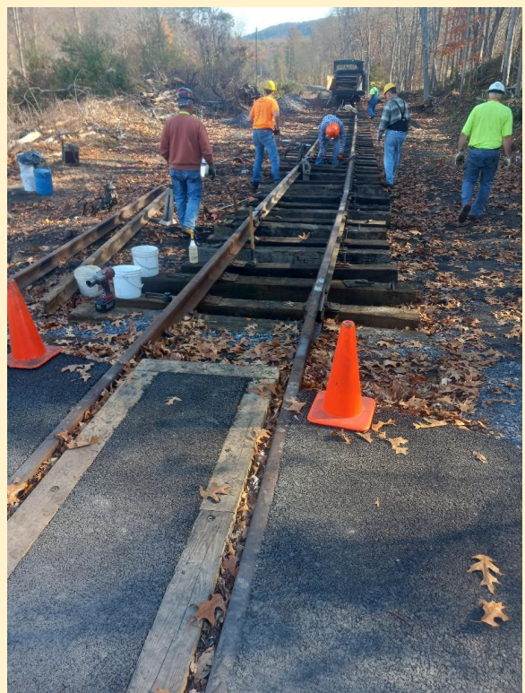
Working on the north side - Oct 31st (G. Tucker photo)
