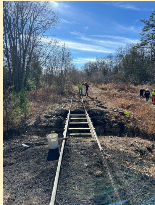
Brushcutting with new bridge - Nov 9th (Roy Burnham photo)
