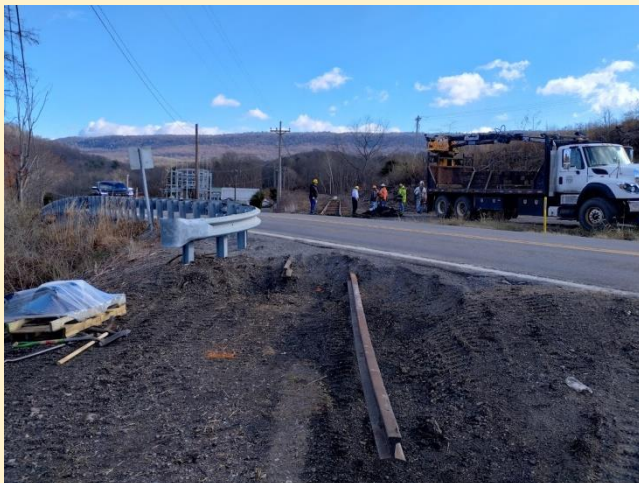
North side of 994 - Dec 3rd (Dave Johnson photo)
