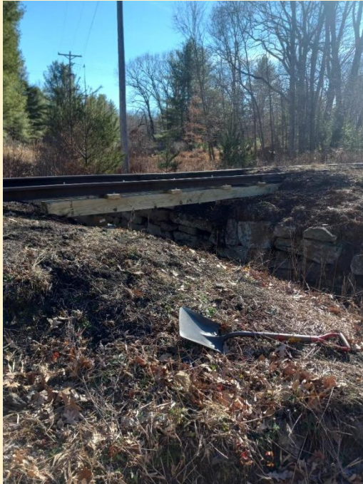
The newest bridge (side view) - Nov 9th (G. Tucker photo)
