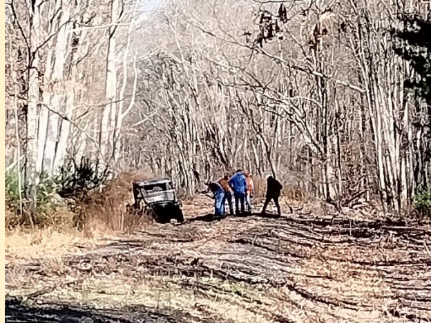
Tie installation north of Wood - Nov 9th (Dave Johnson photo)
